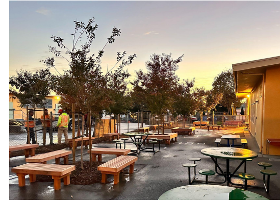
Trees & Asphalt Removal Laurel Elementary
