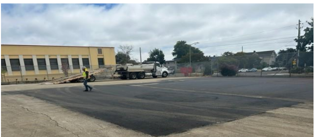
Image 02: Interim Classroom Site Prep
