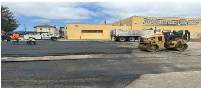
Image 01: Interim Classroom Site Prep
