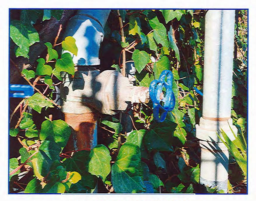
Photo #1 - SOV Leak at BFP
