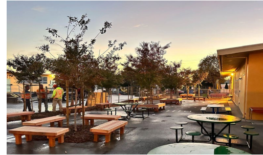
Trees & asphalt removal - Laurel ES
