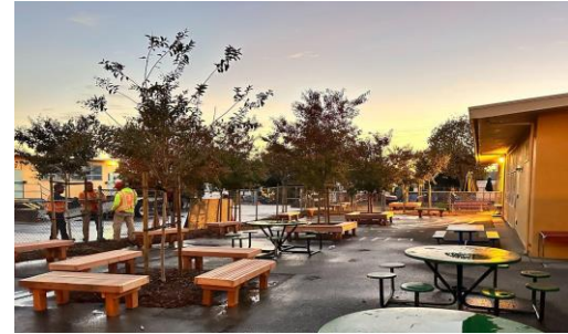
Trees & asphalt removal - Laurel ES
