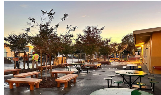
Trees & asphalt removal - Laurel ES
