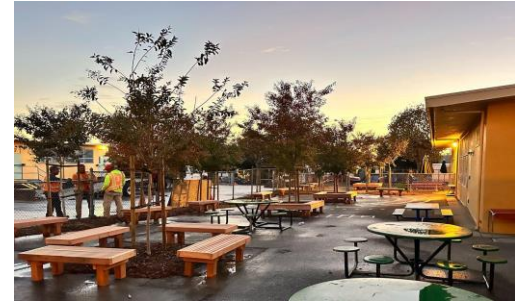
Trees & asphalt removal - Laurel ES
