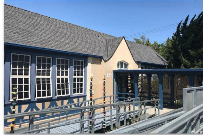
Deferred Maintenance Roof Replacement: Chabot ES, 2025
