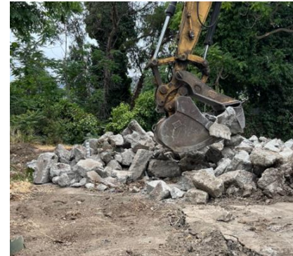
Initial Demolition and Separating Metals, Cement for Recycling (Complete)
