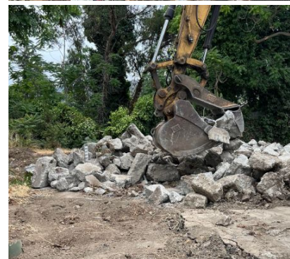
Initial Demolition and Separating Metals, Cement for Recycling (Complete)
