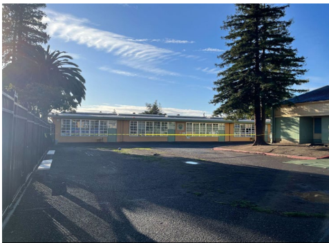
Asphalt Yard - Before Demolition
