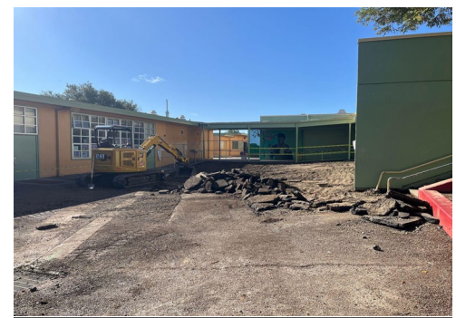
Asphalt Demolition
