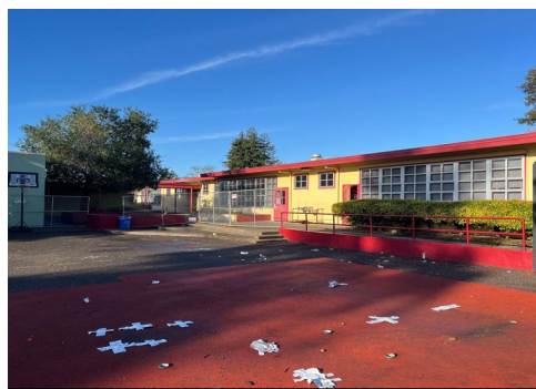
Play Structure Demolition
