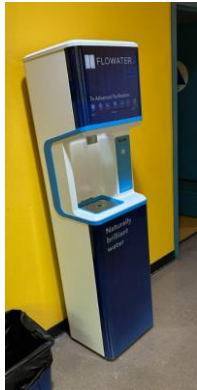
2nd Flowater Unit Installed at Cleveland Elementary
