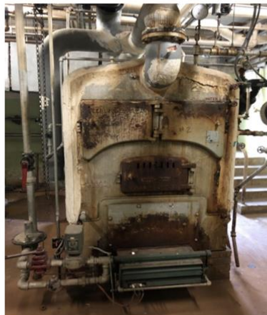
Fruitvale boiler from 1946. It is rusted and only one works
