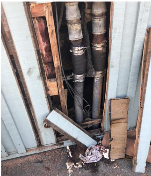
Leaky and rusted boiler pipes at MLK
