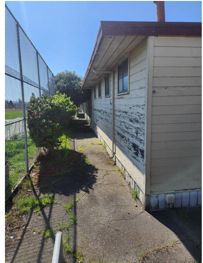
The mural has been graffitied over. The siding on the portable is deteriorating. Grass and weeds are breaking through the asphalt throughout the schoolyard.
