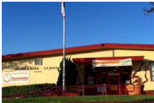
Manzanita Community School Exterior
