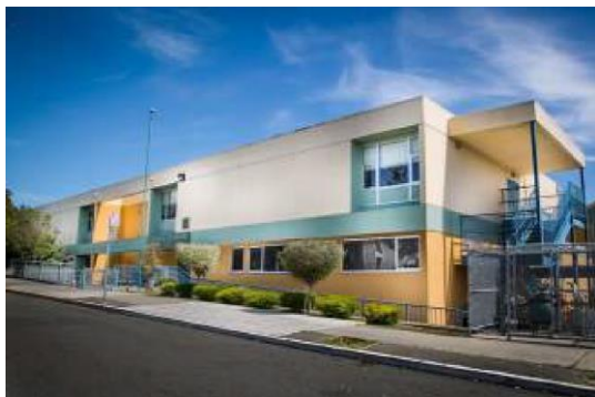
Laurel Elementary School Exterior
