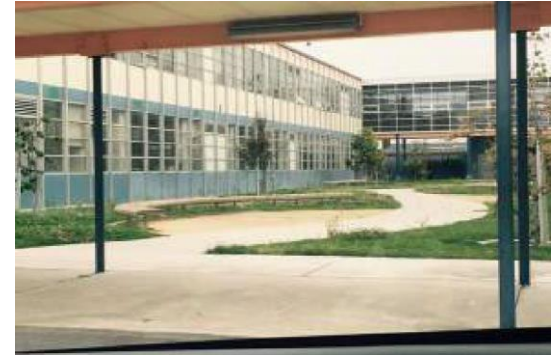
West Oakland Middle School Courtyard
