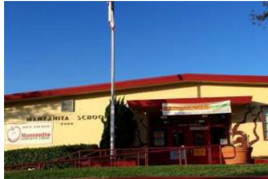
Manzanita Community School Exterior
