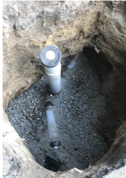
After - Replaced with High Density Polyethylene piping
