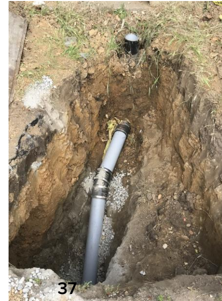
After - Replaced with High Density Polyethylene piping
