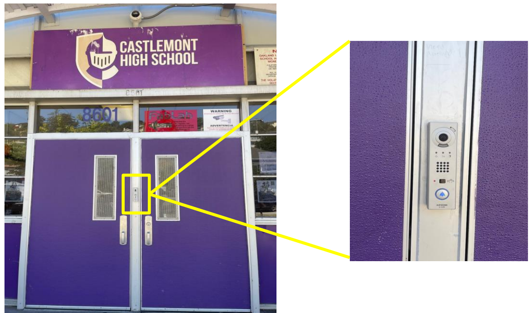
Main entryway area Aiphone IX-DVM door station mounted on center mullion
