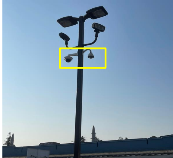
Light pole-mounted security camera
