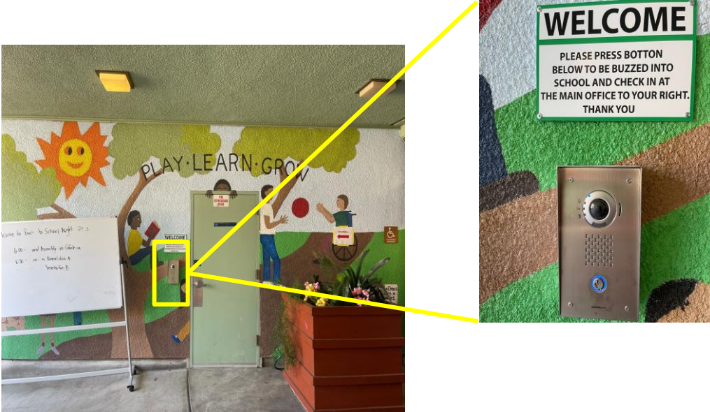
Wall-mounted Aiphone IX-DVF Door Station
