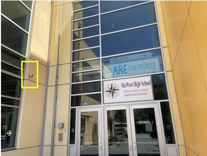
Main entryway area
