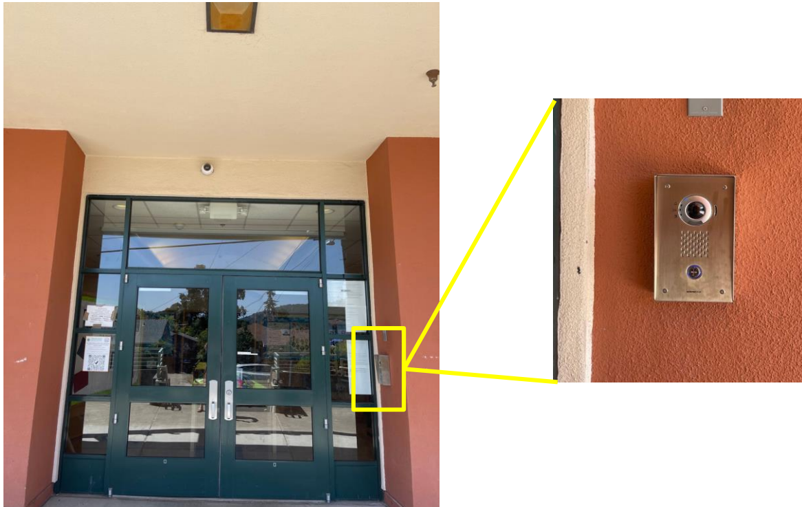
Main Entryway Area
