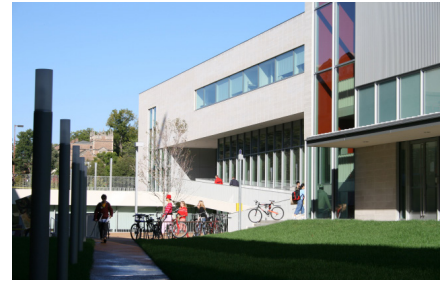
Washington University Sam Fox School for the Arts. SKA assisted Washington University with the master-planning and design of the Sam Fox School of Design & Visual Arts, which include two new buildings and a major renovation of an existing building.
