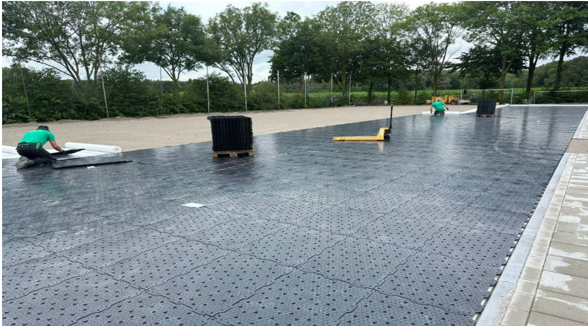
Figure 5 - installation of modular base panels
