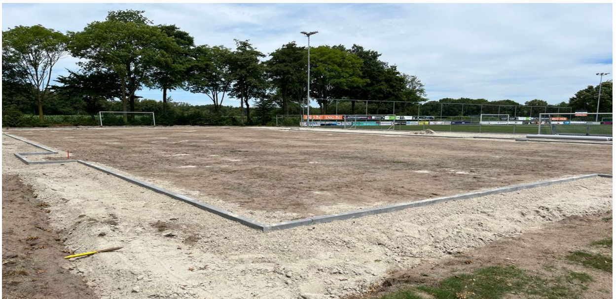
Figure 8 – example of crushed stone base construction
