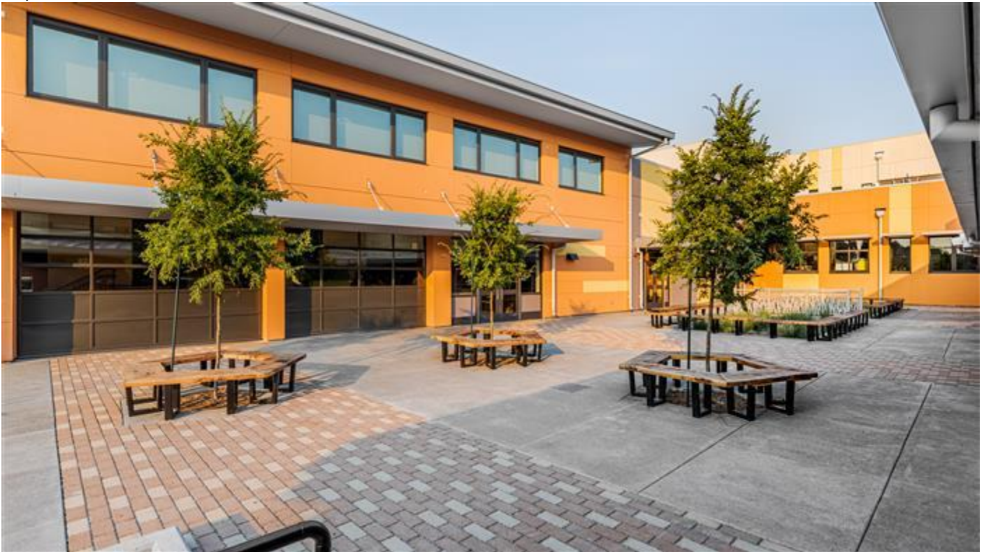
Glenview Elementary Courtyard, part of New Construction Project
