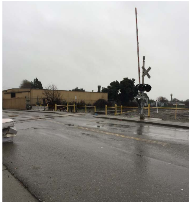
Figure 14: Edes Avenue Crossing, Looking East at South Side of Street
