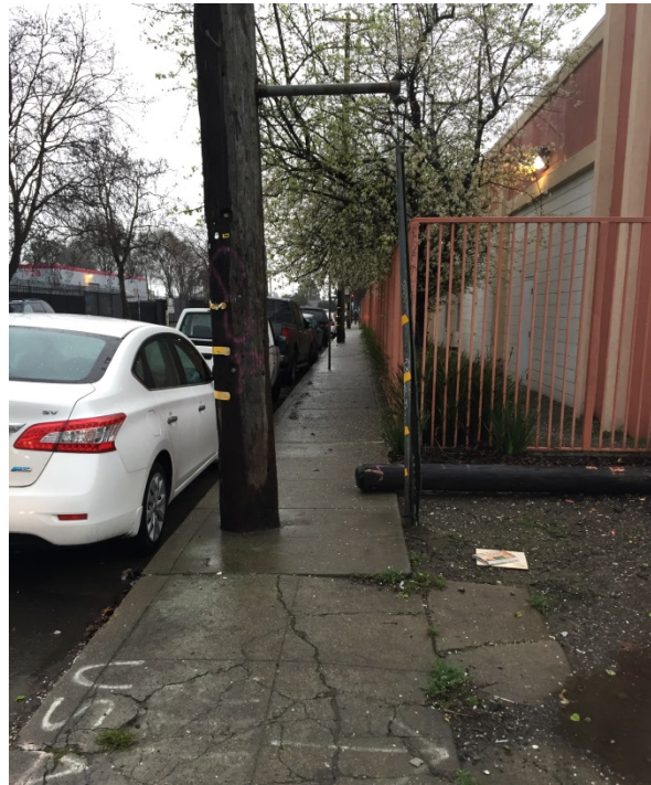
Figure 9: Sidewalk along 105th Avenue, Photo 2
