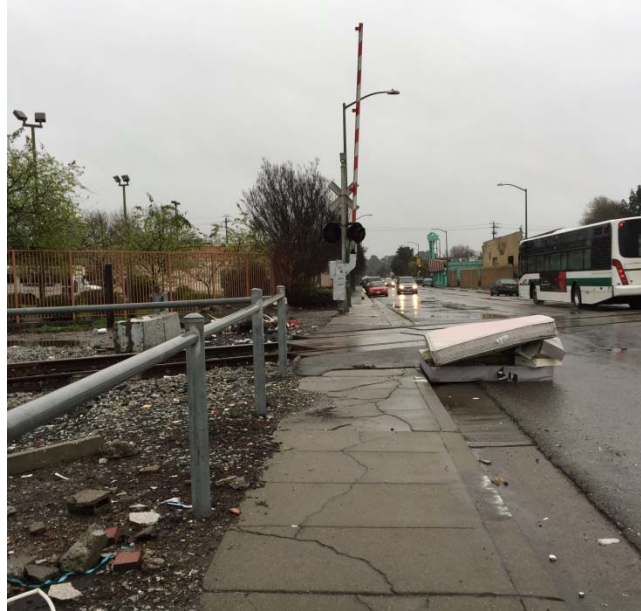
Figure 13: Edes Avenue Crossing, Looking East at North Side of Street
