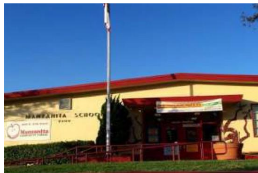
Manzanita Community School Exterior
