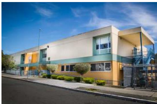
Laurel Elementary School Exterior
