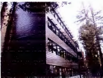
UCSC Biomedical Sciences Facility
