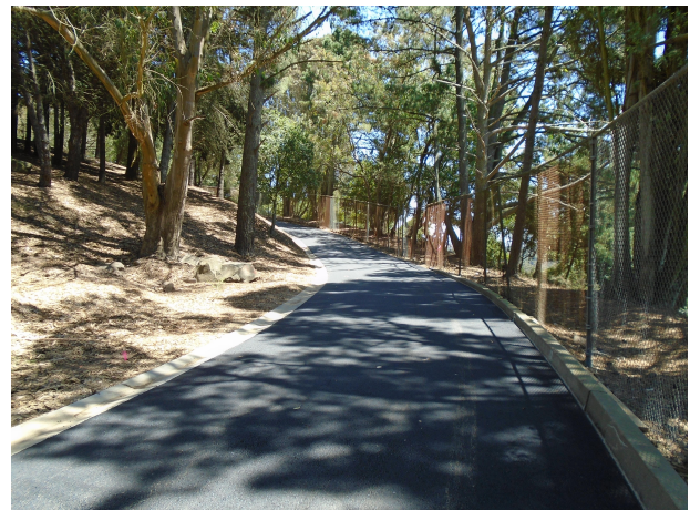
Re-Paved Service Road
