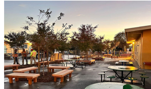
Trees & asphalt removal - Laurel ES
