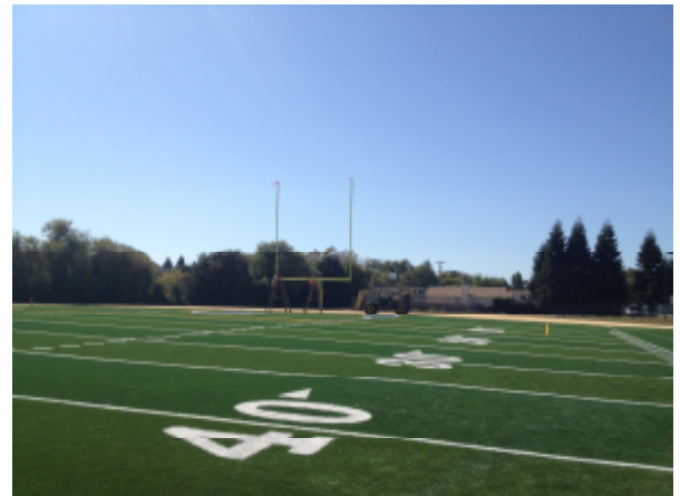
Madison Field Improvements (After)
