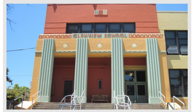
Existing Glenview Elementary Front Entrance Façade to be Retained
