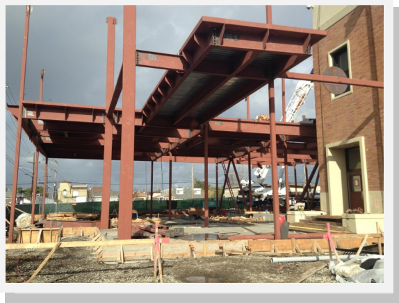
Construction of Two Story Classroom Building
