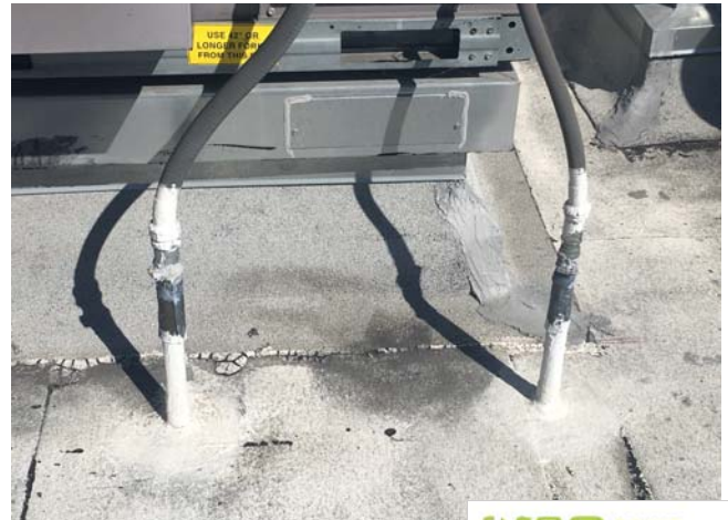
Water Intrusion Mitigation at Roof
