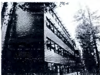
UCSC Biomedical Sciences Facility
