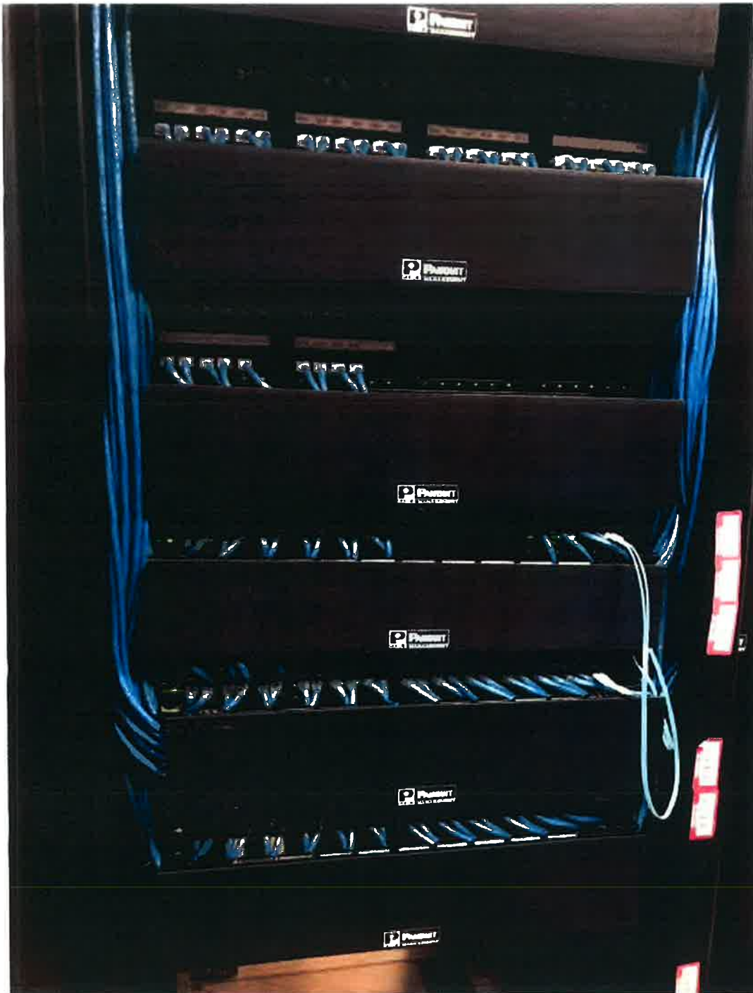
Example 4: Panels labeled, cables are neat, equipment is spaced properly
