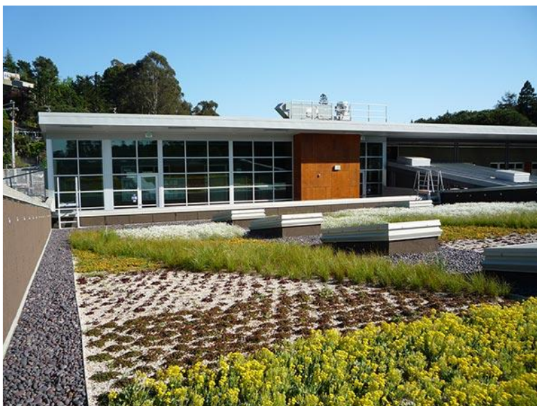
View of Green Roof
