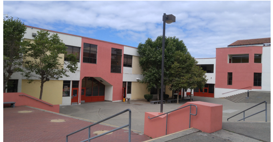
Main Courtyard and Buildings B and C
