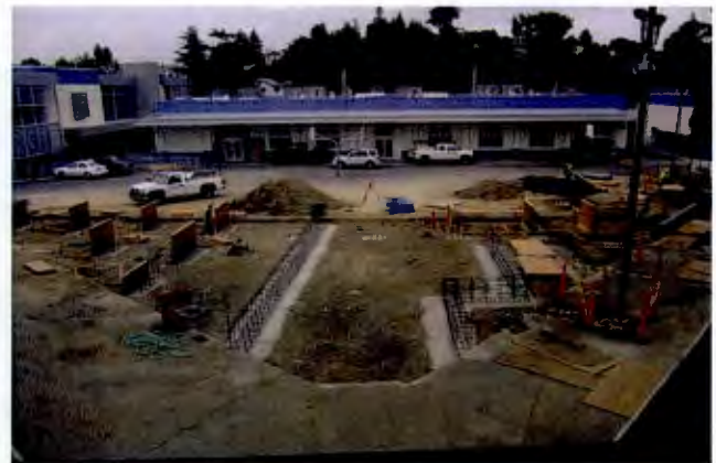
Form-work for benches & piers in the Lower Courtyard
