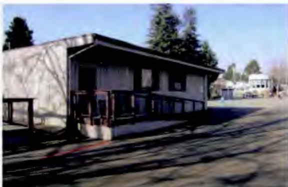
Current science lab will be converted to city library.
