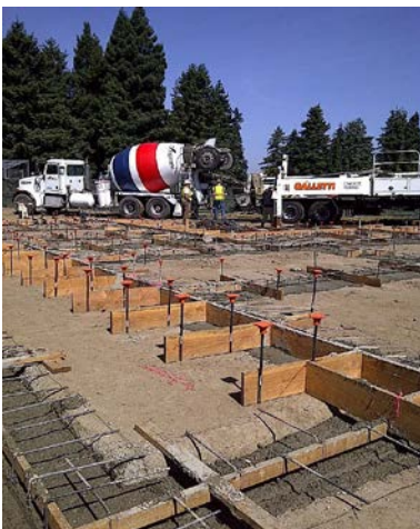
Concrete Poured at Building Footings
