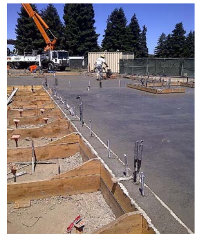
Slab Concrete Poured and Finished
