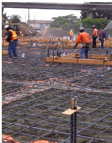
Rebar and Under-Slab Utilities Installed
