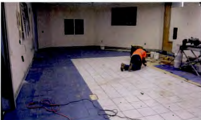
Tile work in the Servery
