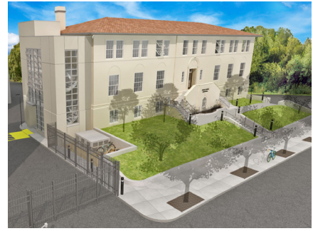
Oakland Unified School District's Educational Leadership Complex is a major renovation of two historic buildings for the District's Central Office Staff. The project scope includes rehabilitation of historic facades, replacement of wooden windows with new historic profile energy efficient aluminum windows, and a new mechanical/electrical/plumbing infrastructure.
