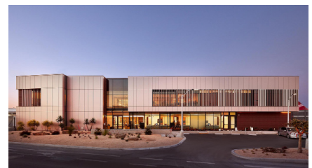
SFO Fire Station 3 is a 20,000 square foot, LEED Gold Certified, essential service facility housing a fire station and training center/ public meeting room prominently located at the Airport's main entry.
