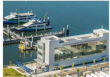
WETA Central Bay Maintenance and Operations Center in Alameda is a 26,000 square foot essential service facility with maintenance shops on the first floor and administrative offices on the third floor. There is a 75 person public meeting room that can be converted into an Emergency Operations
