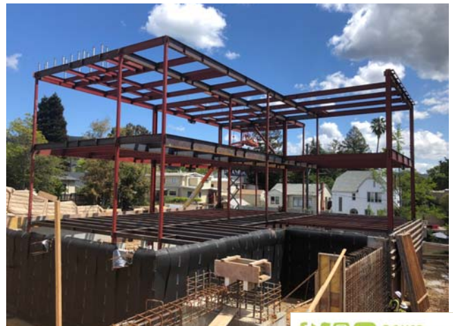
Superstructure basement - set steel
