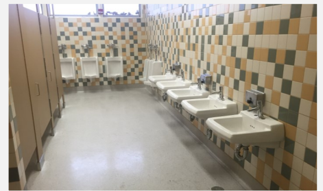
Sobrante Park Restroom Renovation
