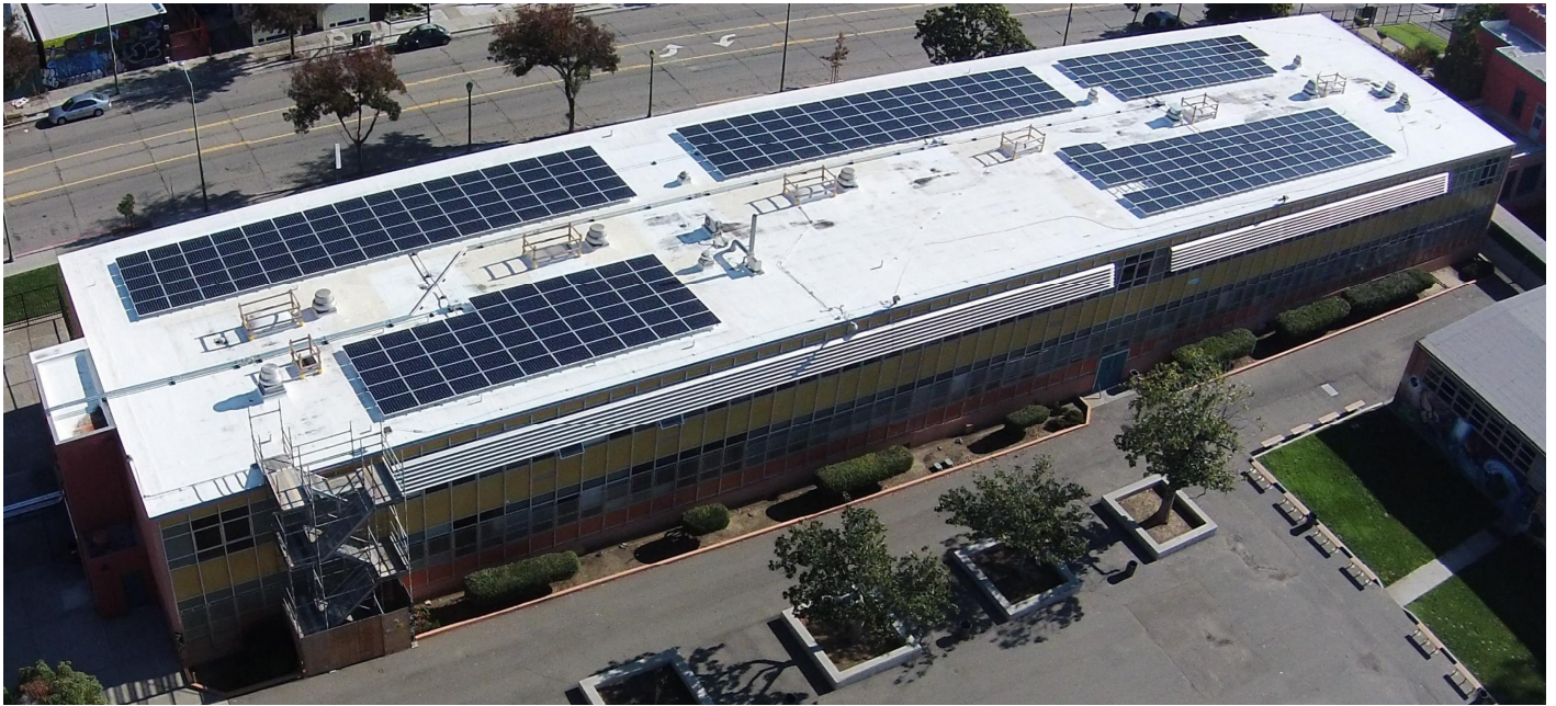
Castlemont High School California Solar Initiative Project
