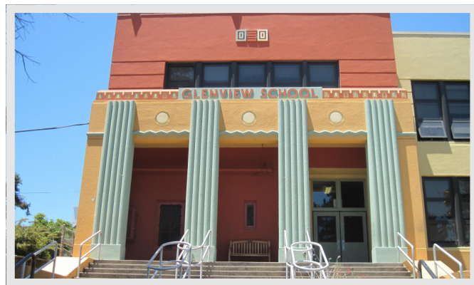
Existing Glenview Elementary Front Entrance Façade to be Retained
