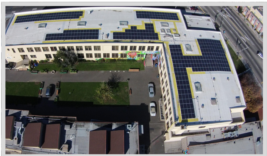
Havenscourt Middle School CSI Project
