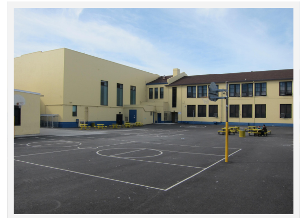
Elmhurst MS Paving Project
