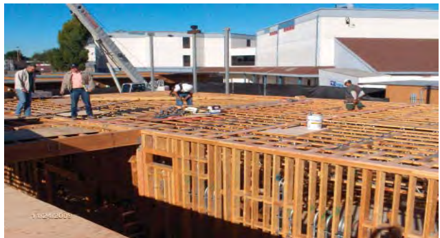
Oakland High School - Framing for New Building
