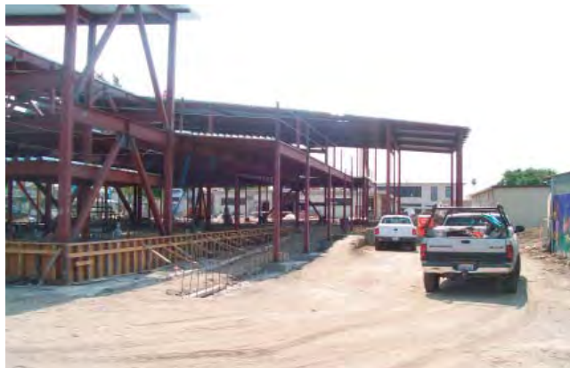
Cox Elementary - Framing for New Building
