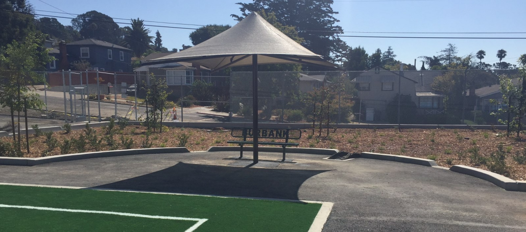
View of New Bioswale & Turf
