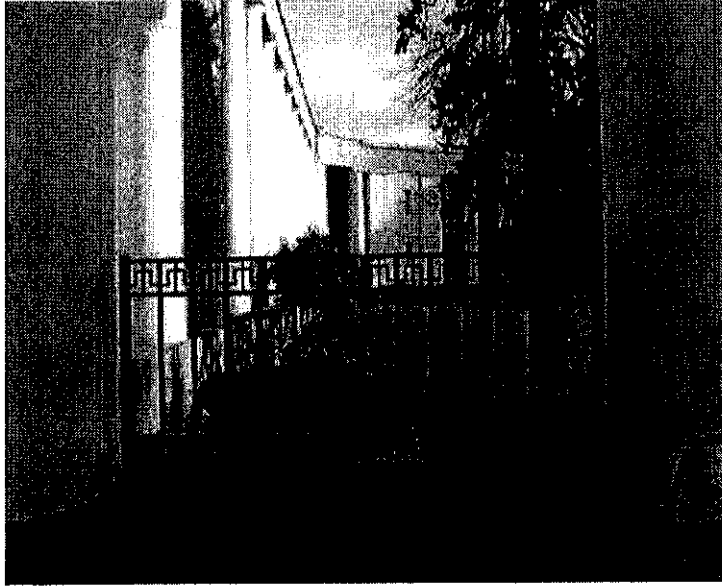
Figure 1. The existing railing at the front landing will be removed to connect the upper landing for the new handicapped access ramp to the front entry. This original historic fabric should be retained and protected in a secure location, and could be used as a model for the new railings for the handicapped ramp. The spacing of individual elements must be changed to meet code.
