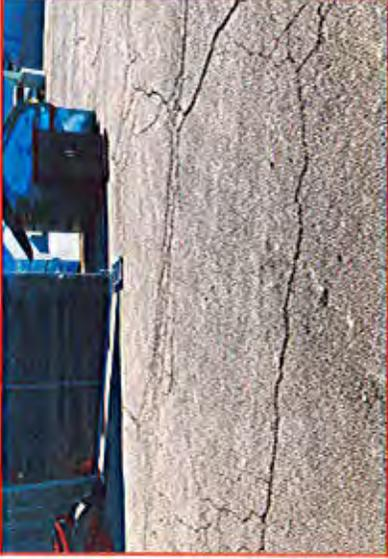
PHOTO 1: CRACKING AND SURFACE WEAR IN THE ASPHALT PAVEMENT, 100% SCALE FOR THE PLAN.
