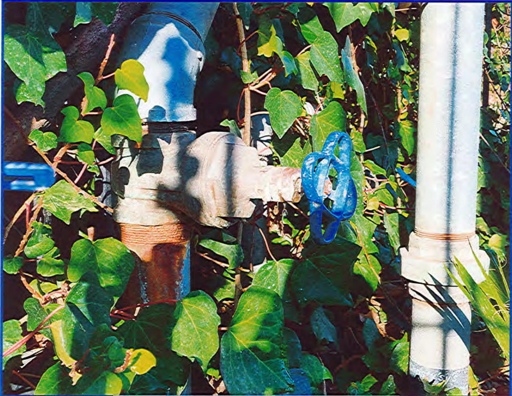
**Photo #1 - SOV Leak at BFP**
