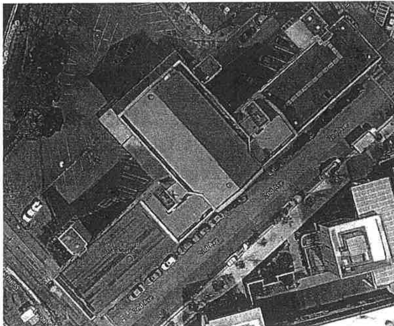
Figure 1. Roof deck location
