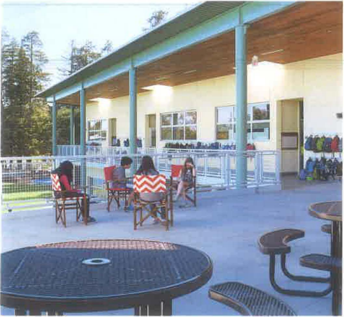
Fairmeadow Elementary School, Palo Alto Unified School District
