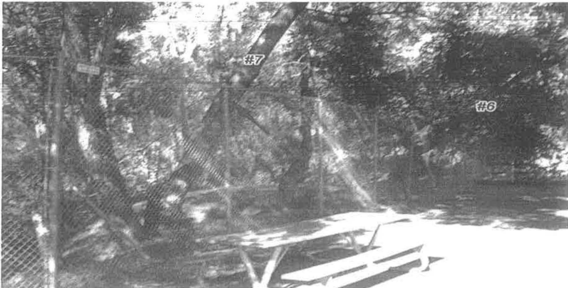
Top photo of Tree #7 shows the severe lean and top-heavy crown. Bottom photo also shows lean and weak crotch at base. Tree poses threat to school grounds (remove leaning section).
