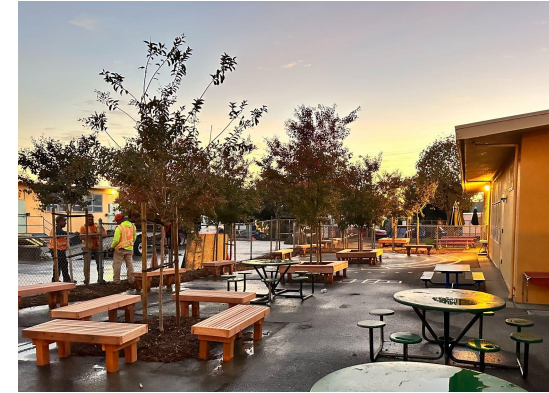
Trees & Asphalt Removal Laurel Elementary
