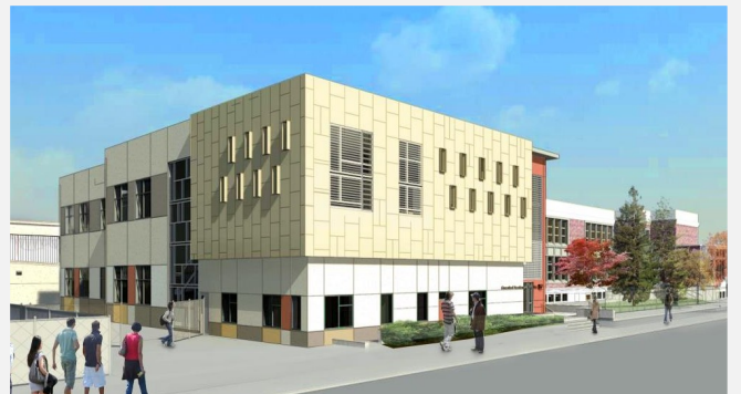
Future Two Story Classroom Building
