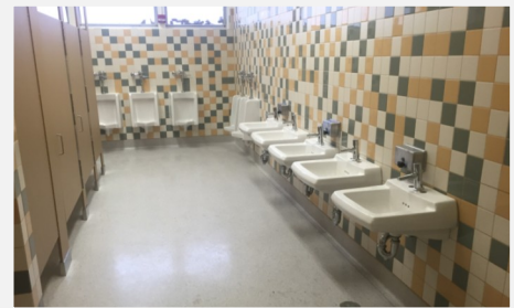
Sobrante Park Restroom Renovation
