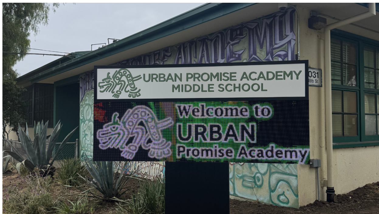
Urban Promise Academy Marquee Installation
