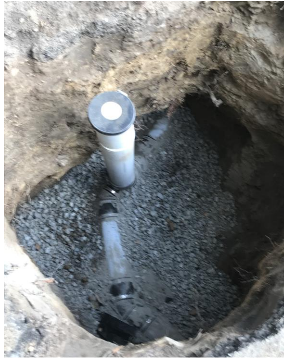
After - Replaced with High Density Polyethylene piping
