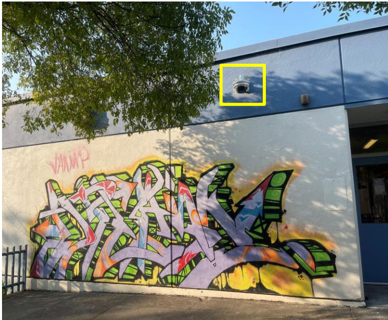
Wall-mounted security camera
