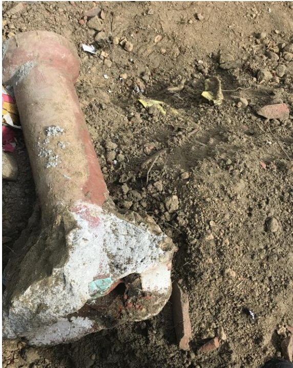
Before - Clay Piping
